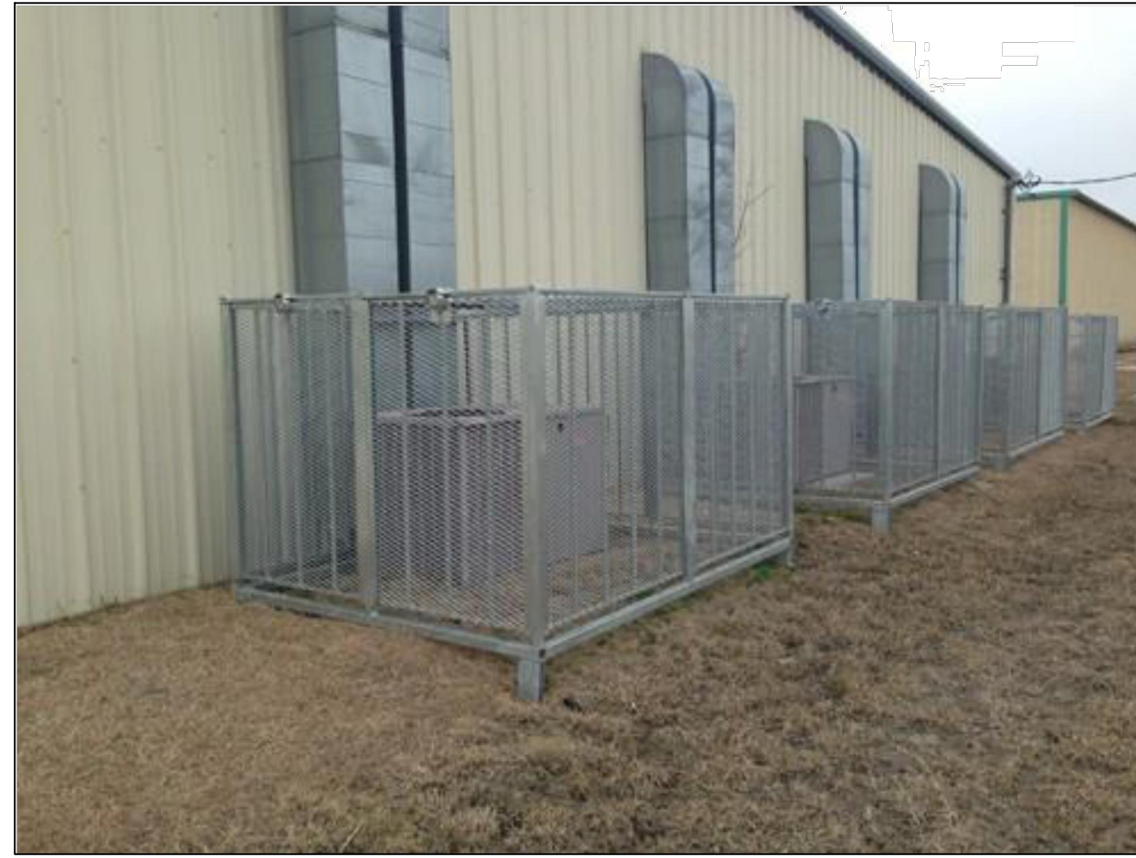
EXAMPLE OF EXTERIOR UNIT SECURITY FENCING
