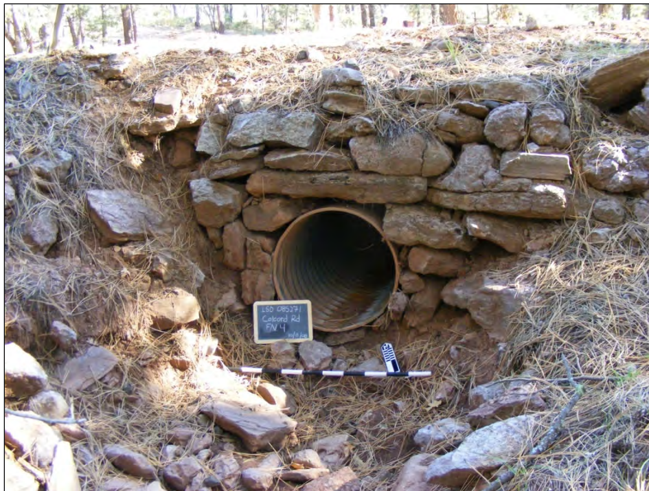
Photograph 5. Feature 2, an example of Type 1B CMP with a dry laid masonry headwall, facing north.
