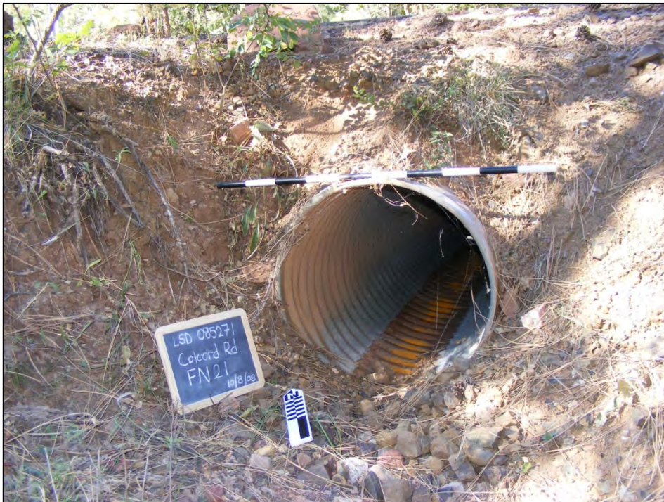
Photograph 4. Feature 9, an example of Type 1A CMP, facing south.
