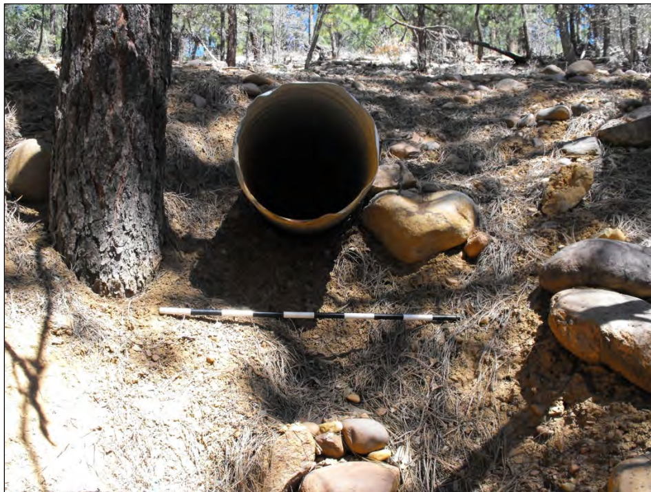
Photograph 3. Feature 58, an example of Type 1A CMP, facing north.
