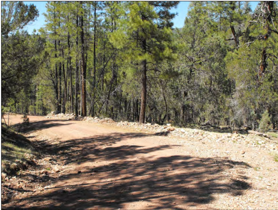
Photograph 1. Photograph of the historic Colcord Road showing cobble and earthen berms along the northern shoulder of the roadway, facing north.
