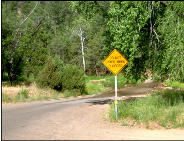
FIGURE 3-11. EXAMPLES OF ROADWAY SAFETY ISSUES
