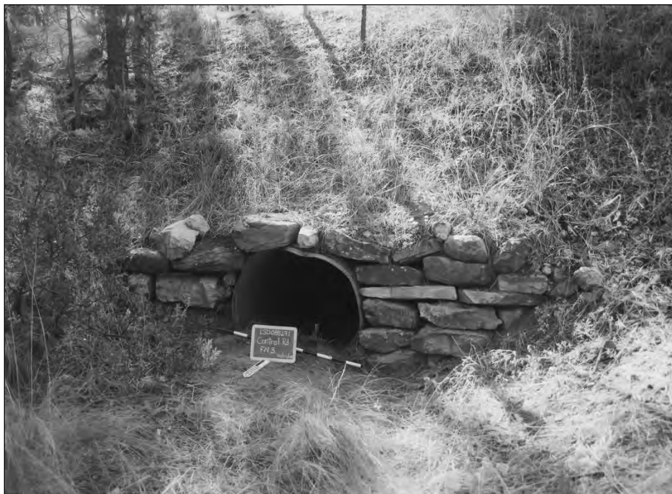
Photograph 2. Feature 3, a dry-laid Type 1B feature with a single CMP, facing southeast.
