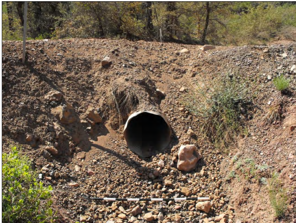
Photograph 1. Feature 235, an example of a Type 1A culvert, facing northwest.
