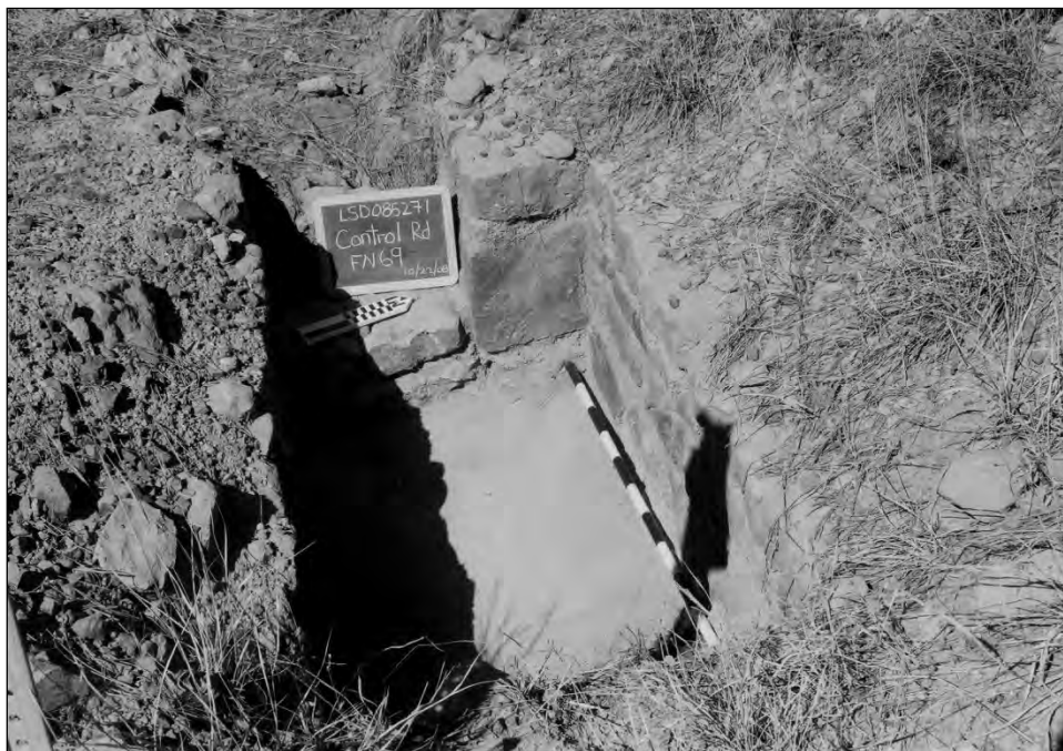
Photograph 6. Feature 54, an example of a Type 1C feature with a prepared concrete floor, facing west.
